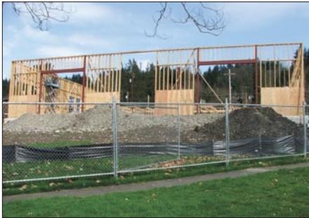
The new Vernetta Smith Chehalis Timberland Library under construction.
