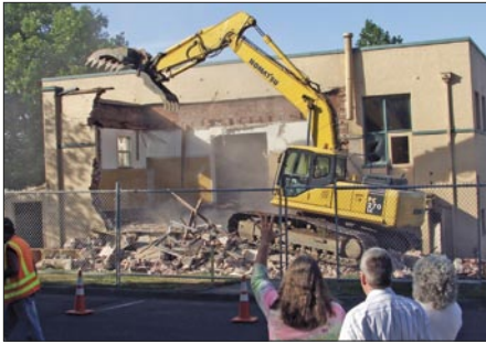
Chehalis Timberland Library demolition.
